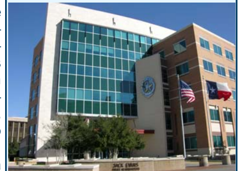
The Dallas Police Headquarters consolidated 1,300 police employees previously spread through multiple sites.
