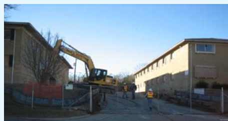
Workers begin demolishing the Chateau Crete Apartments
